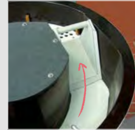
Manually inserted separation gate
