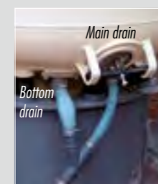
Combined media unload plug with effluent drain (main drain)
